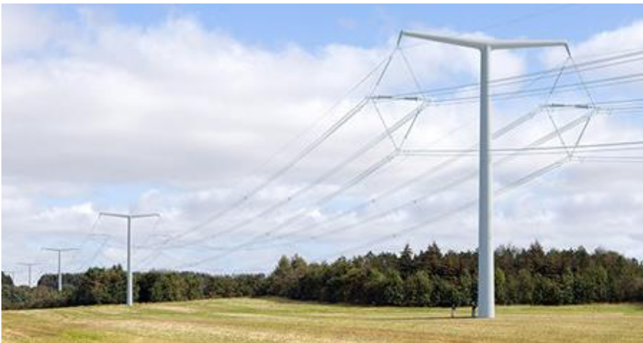
Figure D.25 : National Grid's T-pylon
