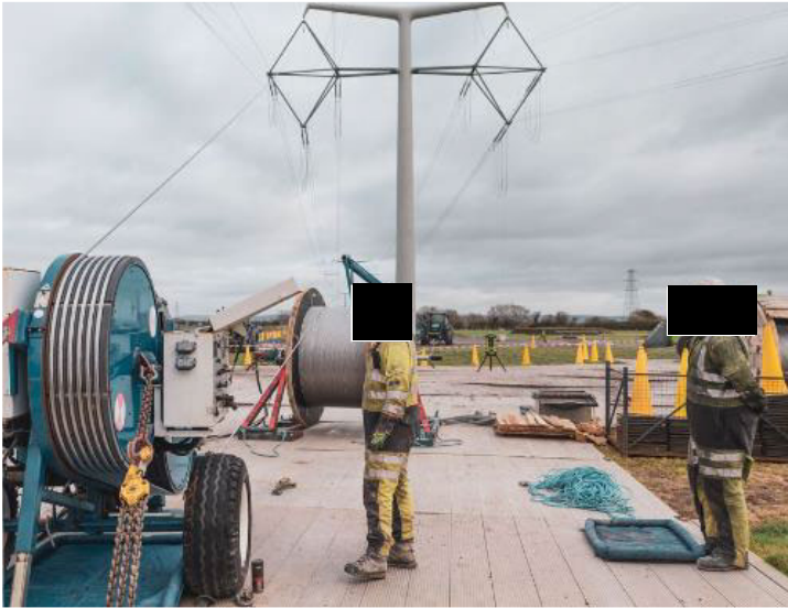
Figure D.17: Stringing site during T-pylon line construction
