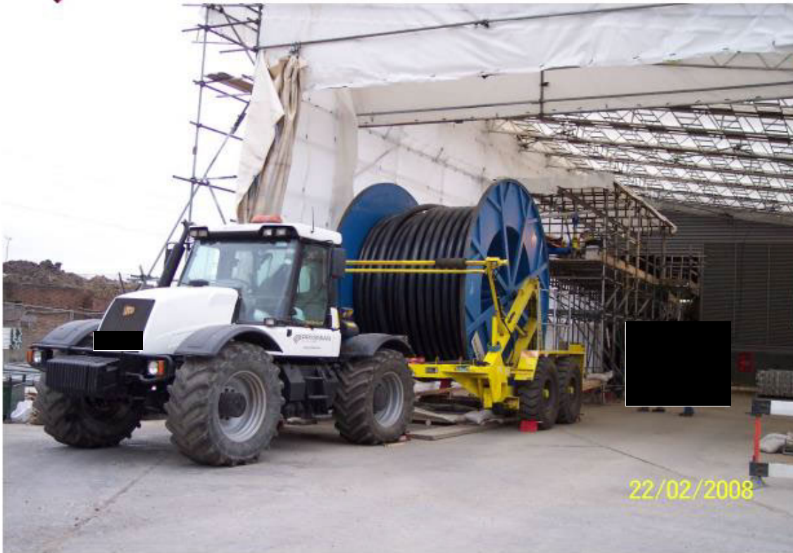
Figure F.8: Cable winching from drum
