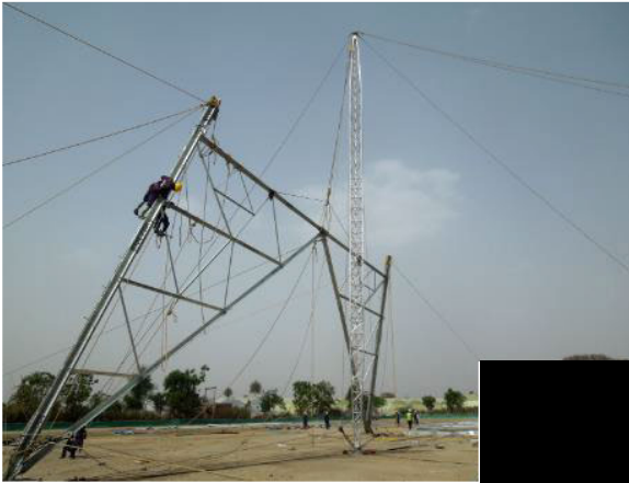
Figure D.15: Erection using derrick pole
