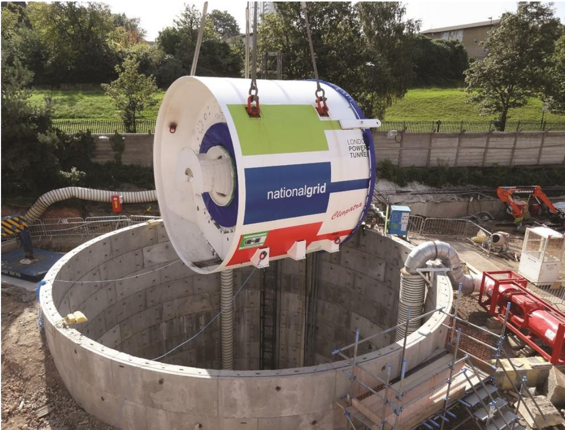
Figure F.2: Tunnel shaft insertion
