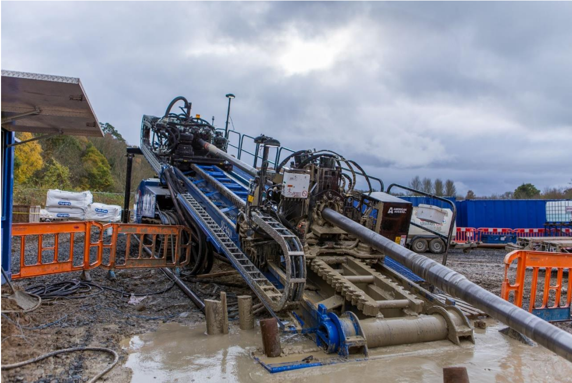
Figure E.8: HDD rig
