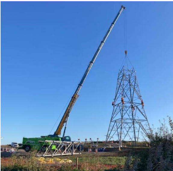
Figure D.14: Crane erecting tower sections
