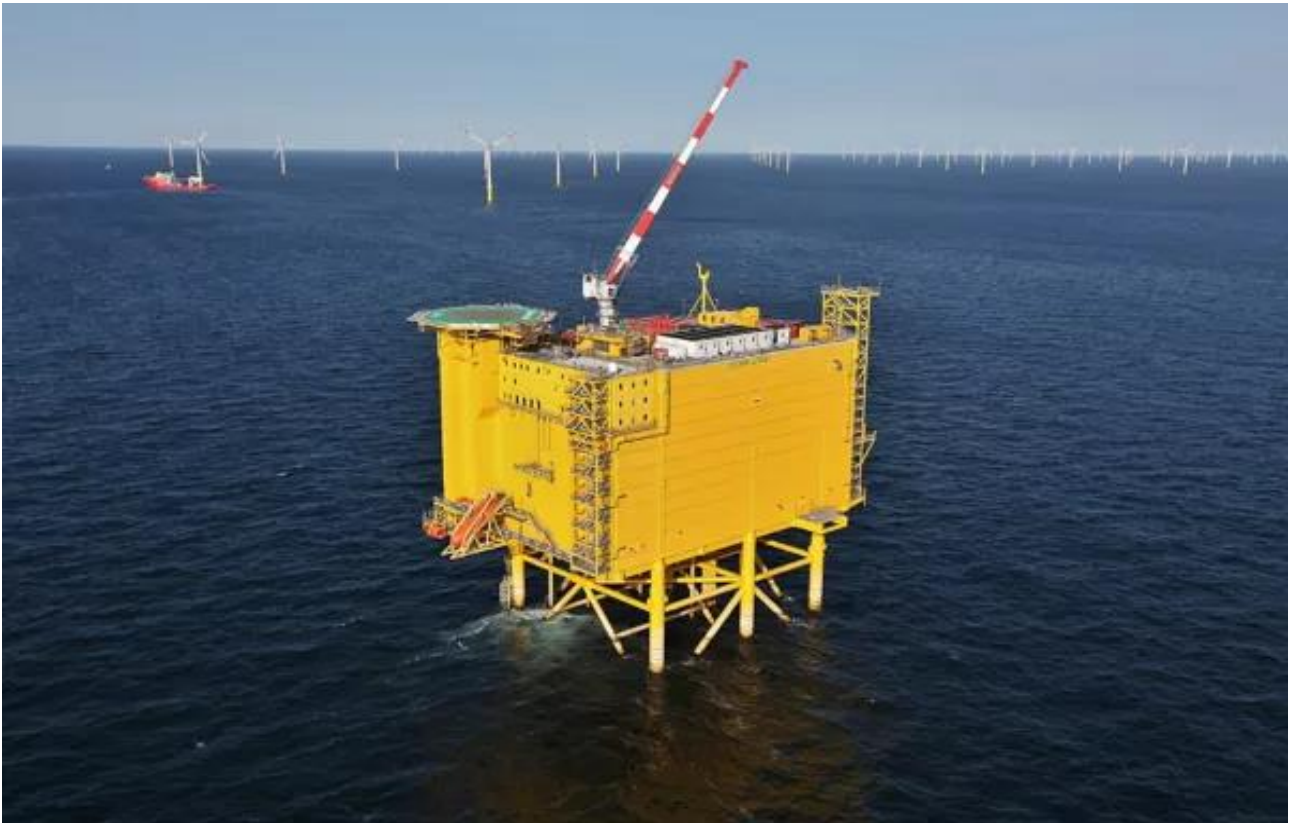
Figure G.5: DoIWin Alpha offshore platform
