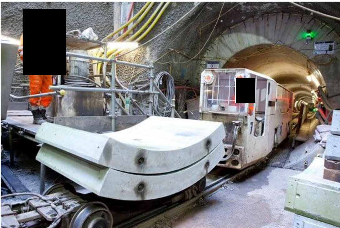
Figure F.15: Rail installation for London power tunnels 2
