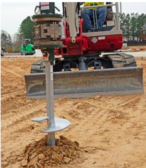
Figure D.13: Excavation for augured foundation
