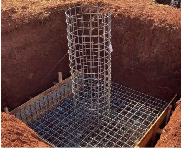
Figure D.12: Pad and chimney foundation
