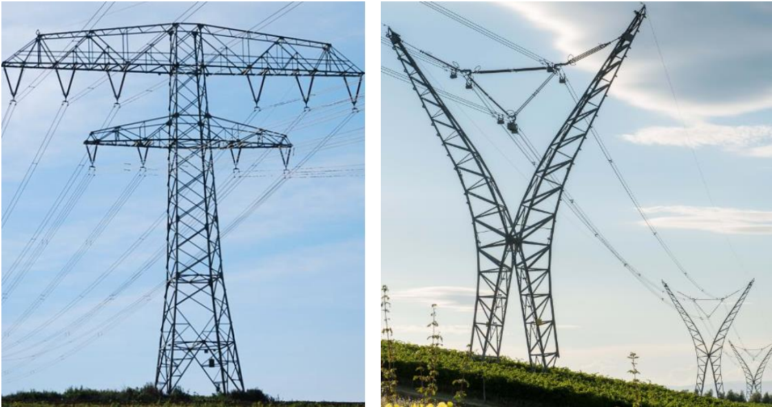
Figure D.24: a) 420 kV line with V-strings, b) 380 kV line in Italy
