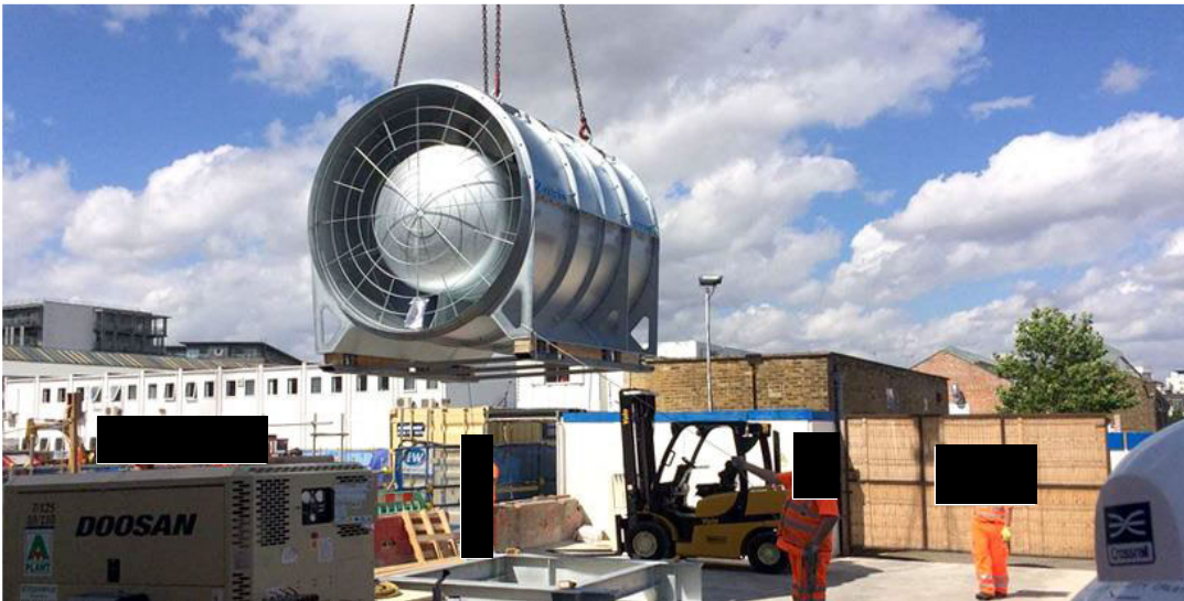
Figure F.5: Tunnel ventilation system installation
