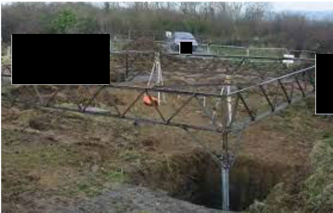
Figure D.11: Foundation setting template
