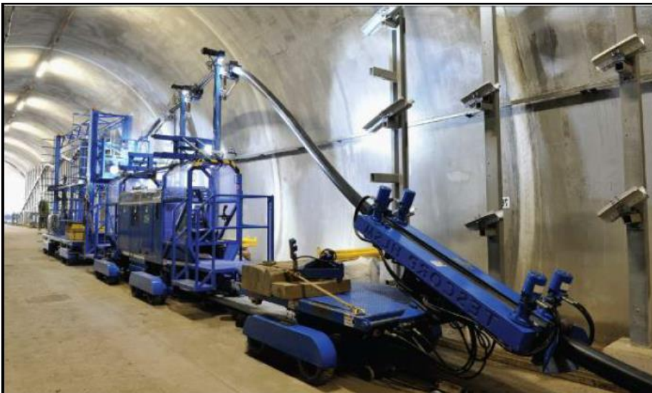
Figure F.10: Automated tunnel cable installation machine
