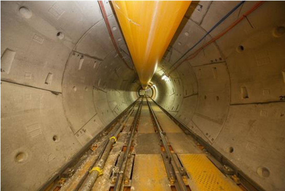
Figure F.7: Tunnel showing outer segments
