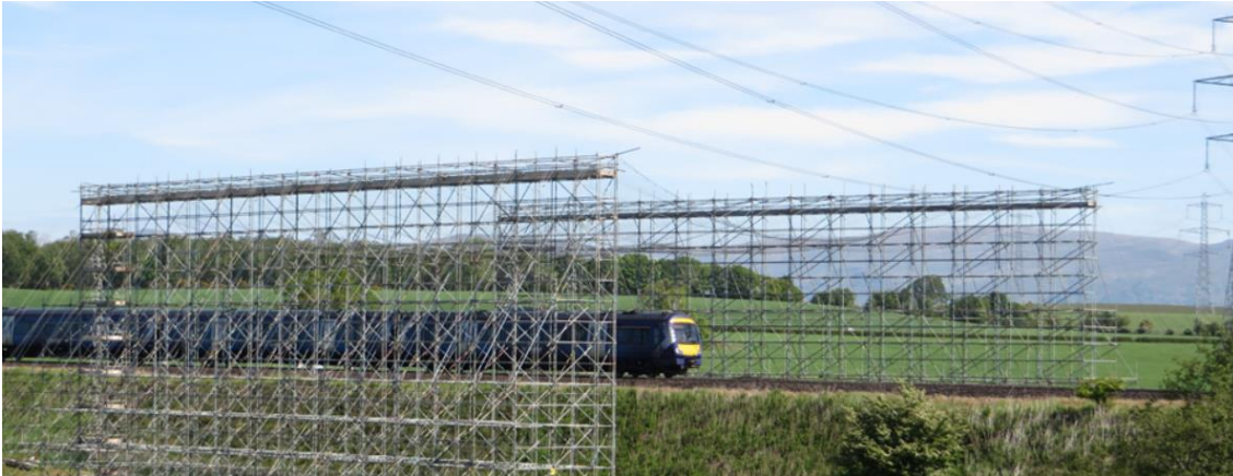
Figure D.10: Scaffold protecting railway line
