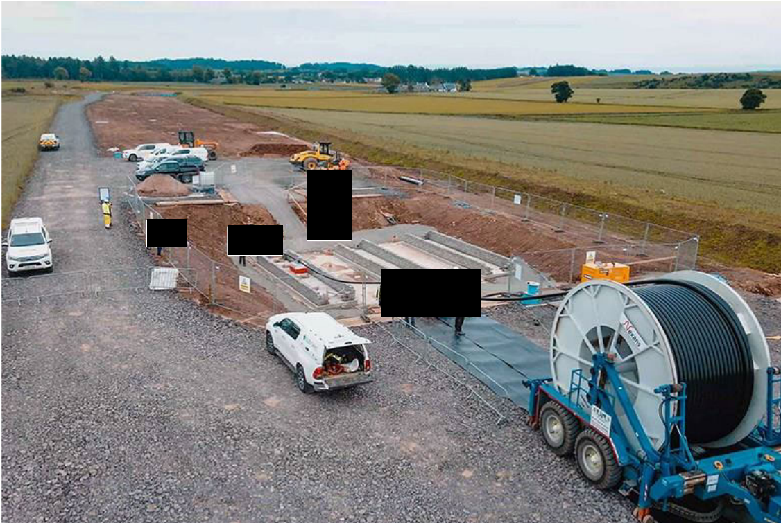
Figure E.7: Cables being pulled into ducts at joint bay location
