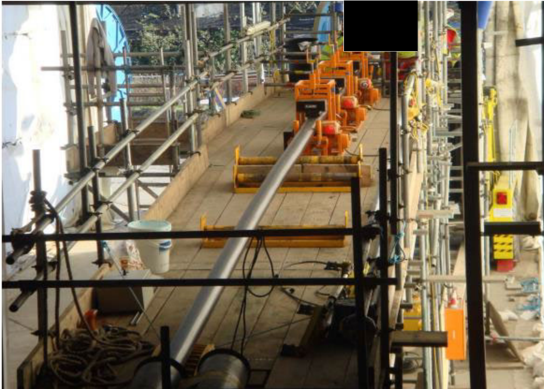
Figure F.9: Cable being lowered into tunnel
